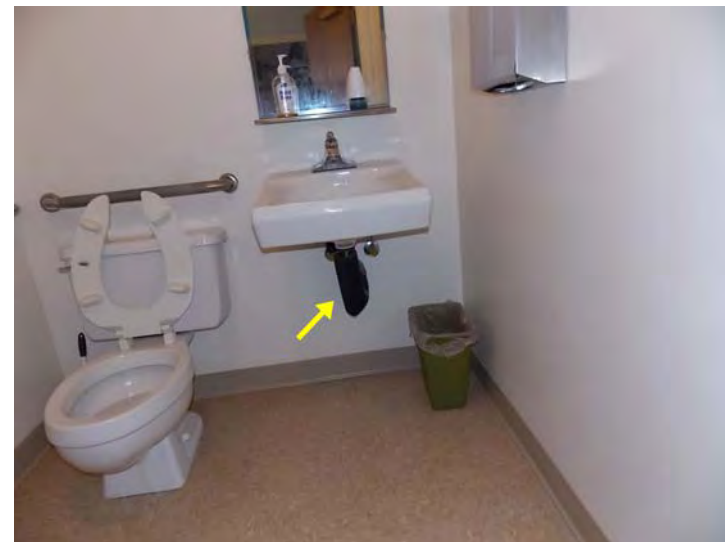
One of the public restrooms, note the insulated drain line.
