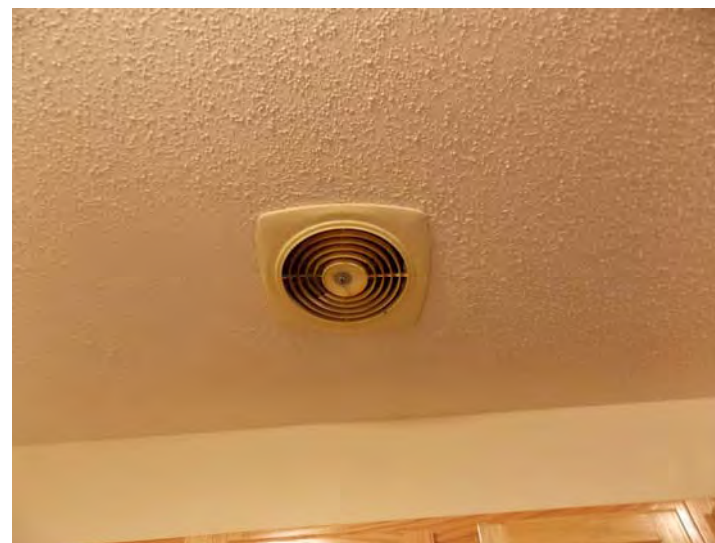
A typical kitchen ceiling exhaust fan.
