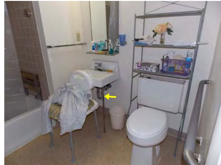
This is one of the accessible bathrooms; a grab bar behind the toilet and drain line insulation (arrow) should be added.
