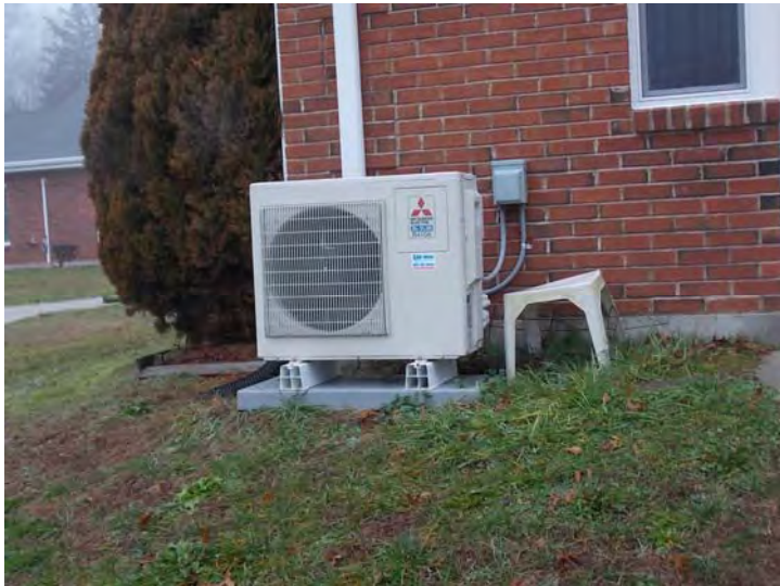
One of the air-cooled heat pumps.
