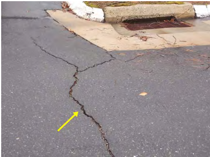
A close-up view of a cracked asphalt section.
