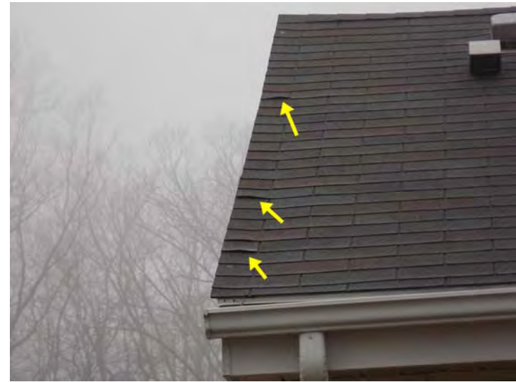
An example of several lifting roof shingles.
