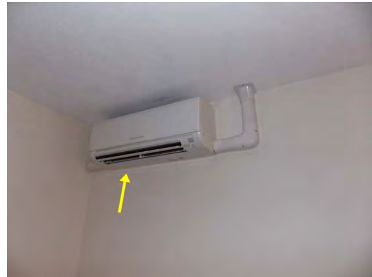
This is one of the heat pump terminal (fan coil) units.
