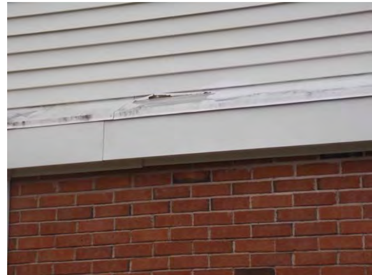
Peeling paint on an aluminum trim section.
