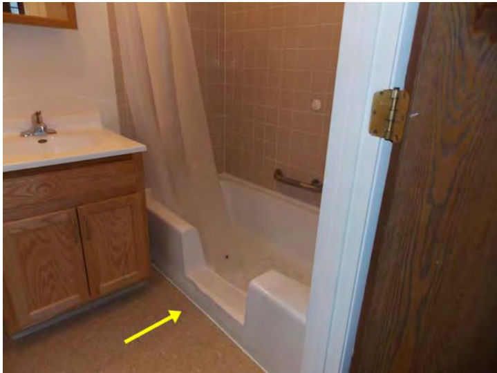
Bathtubs are being upgraded with tub cuts.
