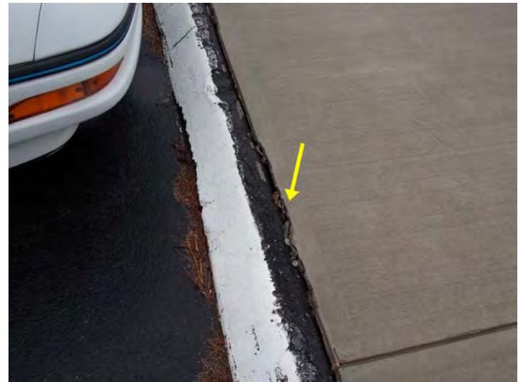
A chipped edge of a walkway section.
