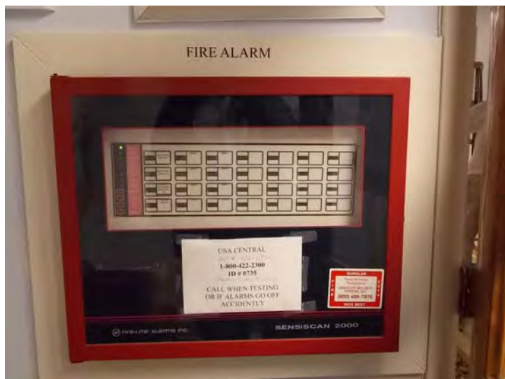
The central fire alarm control panel is located in the community building.
