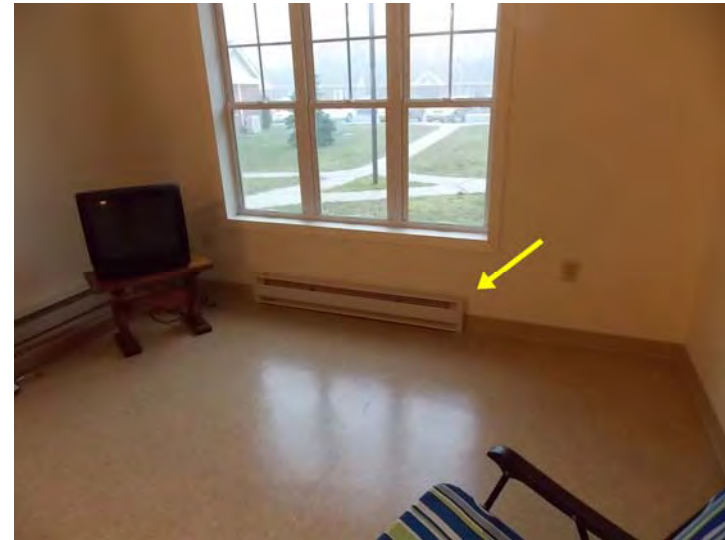
Electric baseboard heat augments the heat pump output.
