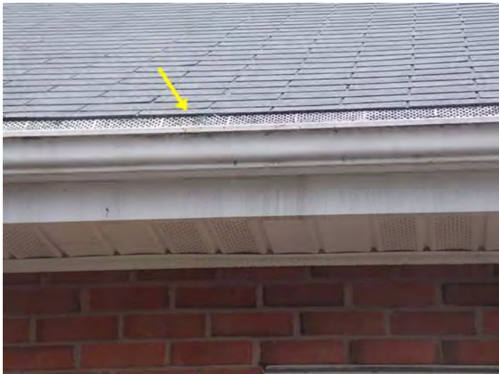
This gutter guard helps to keep leaves and debris from accumulating in the gutters.
